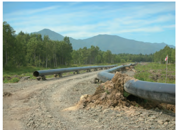
Photo 6. Pipe line under construction.
